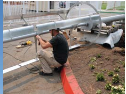
4. Assemble Rotor
