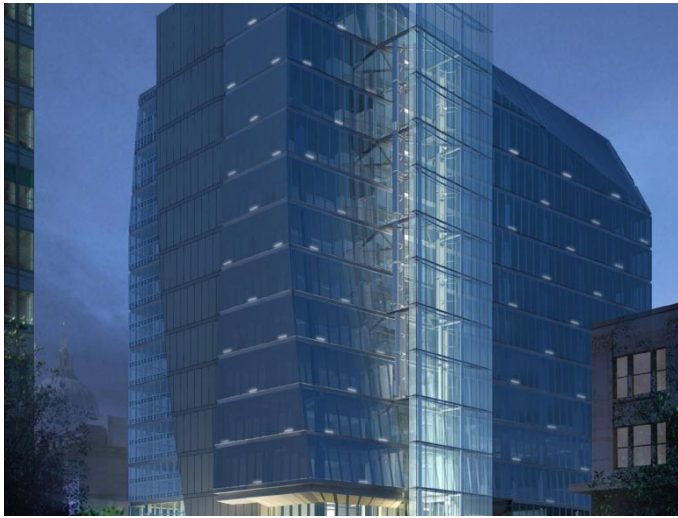
PUC Building, San Francisco
